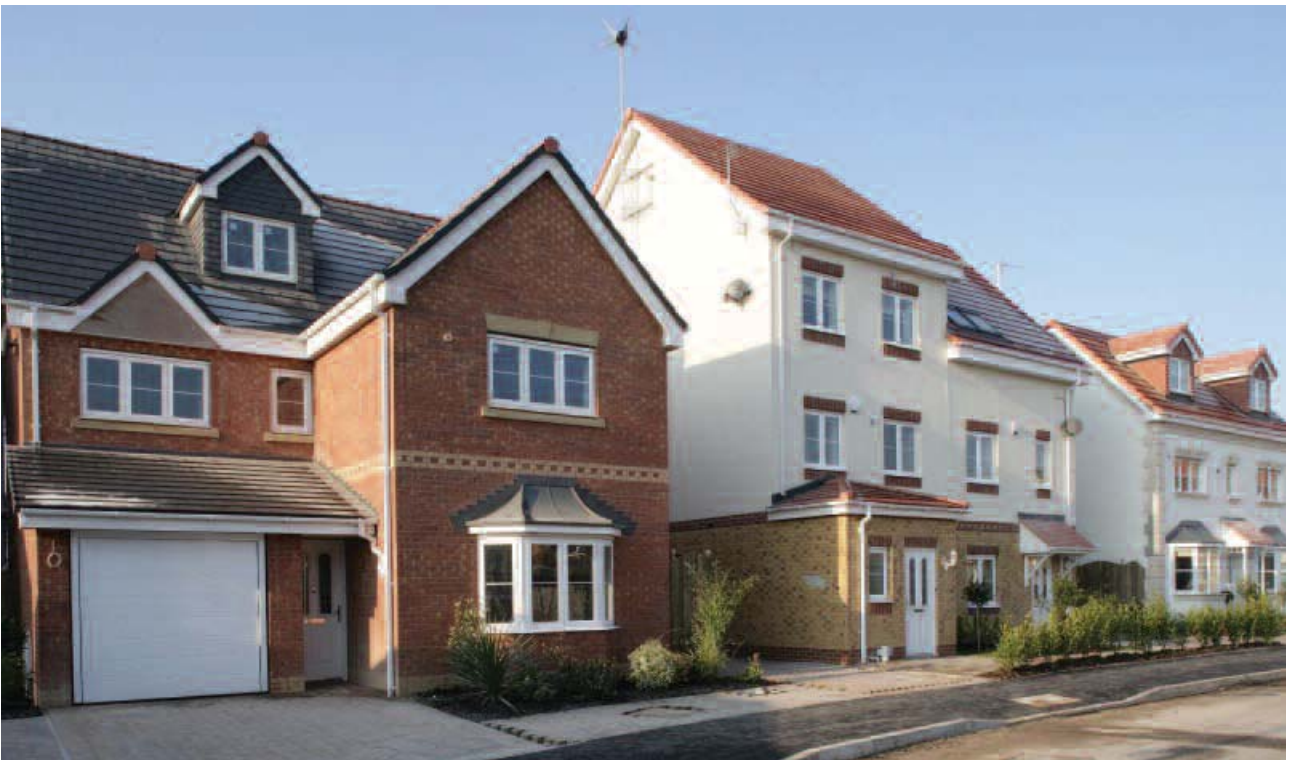
Building for the future: The Living 1 Project at Irlam, Manchester
