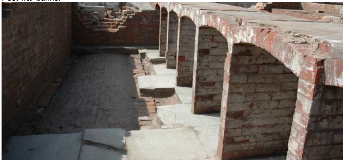
Cellar and basement of the New Hall
