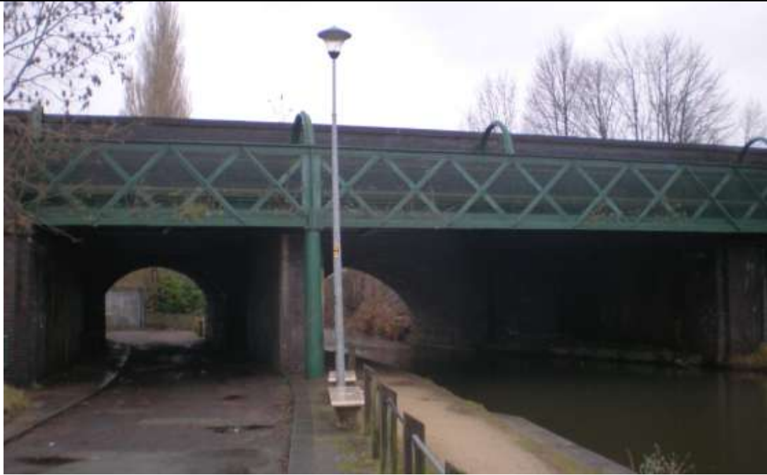
View from the south.
