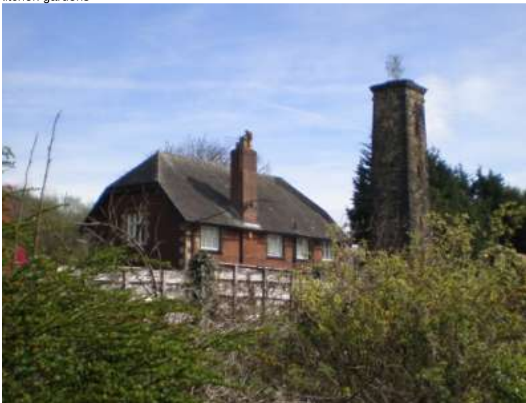
Boiler house and underground stables
